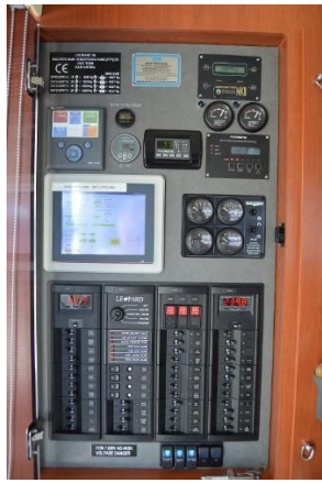
Custom Electrical Panel
