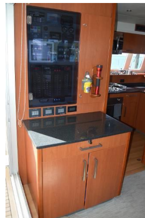
Electrical Panel and Entry Locker
