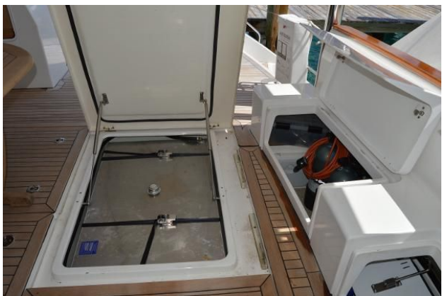
Additional Fuel Tanks
