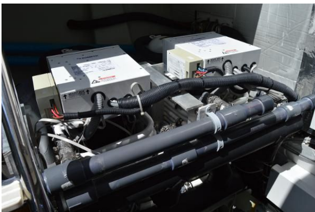
Dometic Chiller System
