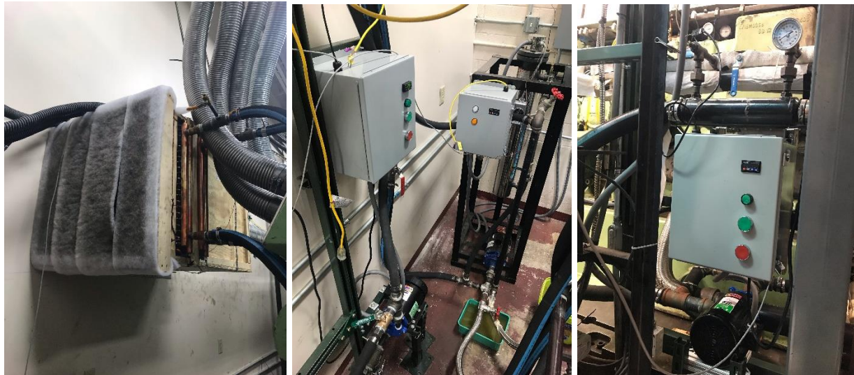
Figure 7: The intake air plenum (left), the heating and cooling fluid controllers and pumps (center), and the fuel cooler with controller and pump (right)
