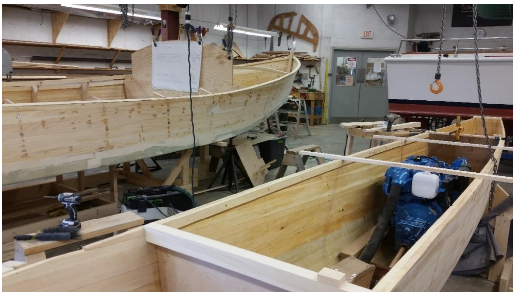
Figure 9: Construction progress showing diesel engine in main hull.
