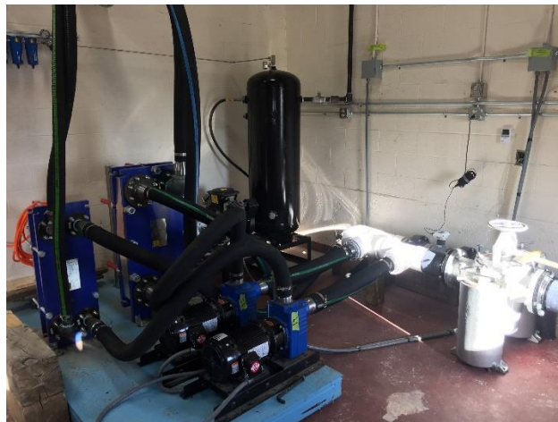
Figure 8: The salt water cooling system
