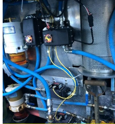
Figure 1.2: Starboard switching valves, fuel filters and flow meters on board Quickwater .
