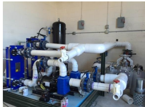
Figure 10: Seawater cooling and air start systems
