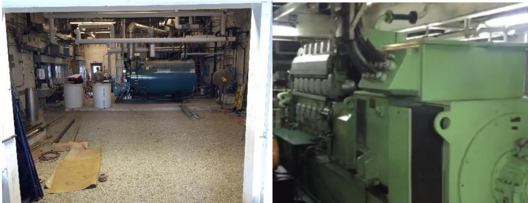
Figure 14: (Left) Andrews Hall on MMA campus, the location of the medium speed engine lab under construction, (Right) Wartsila 6L20 diesel generator set on order for the lab
