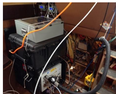
Figure 6: CEM system on Quickwater
