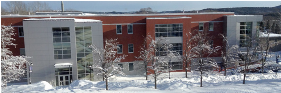
The new ABS Center is partially supported by the Harold Alfond Foundation. Photo by L Stone.
