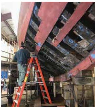
Spiles being hammered into frames and plank replacement during the hull restoration in 2018.
