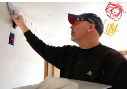
Shawn Heath, Building and Grounds Tradesworker II, a member of the Facilities team renovating the Wyman House
